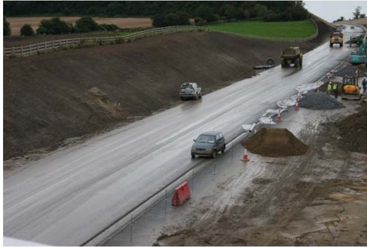
Works going ahead on the N9 motorway
