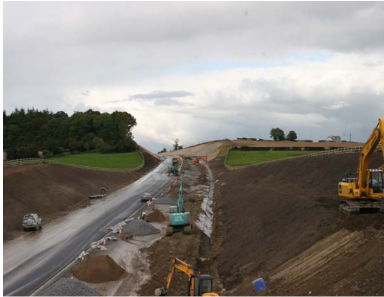
A view of the continuing works from the Russelstown overpass
