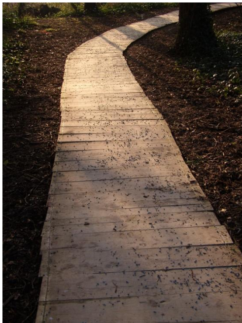
Figure 16: Example of the walkways.
