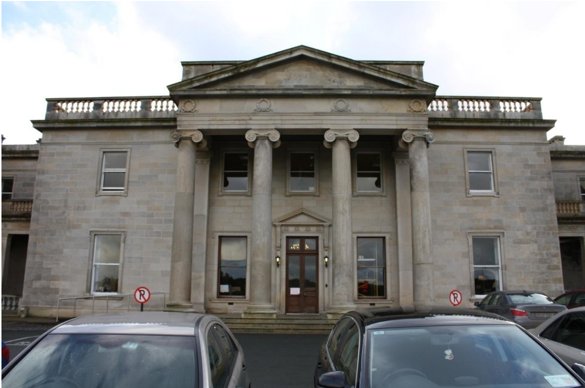
Figure 13: The front façade of Oak Park house
