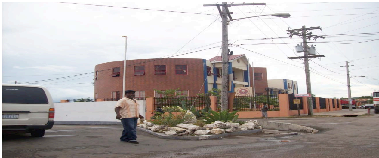
Figure 9 A proud resident walks past the renovated fire station. Photo courtesy of Alcia Bromfield
