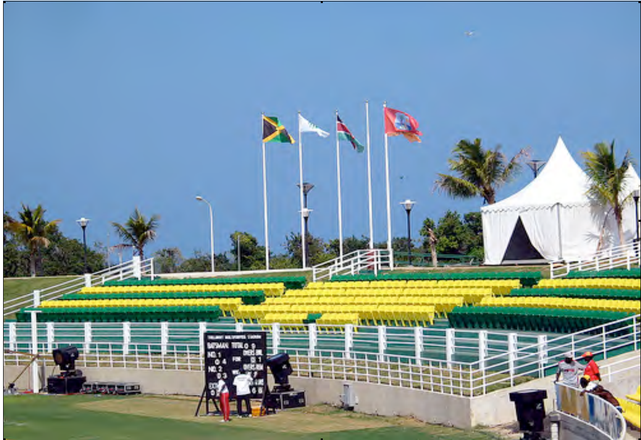
Figure 1 Building the Trelawny multipurpose stadium. Photo courtesy of www.cwc.org
