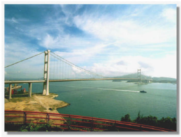
Tsing Ma Bridge
