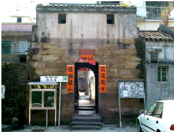
Entrance Tower of Ma Wat Wai
